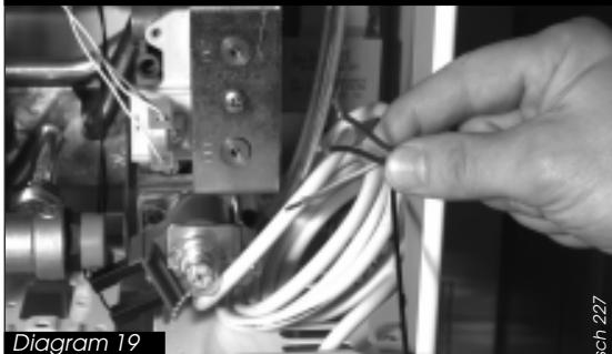
The mains electrical cable is supplied with the boiler. It is coiled and tucked inside the boiler
